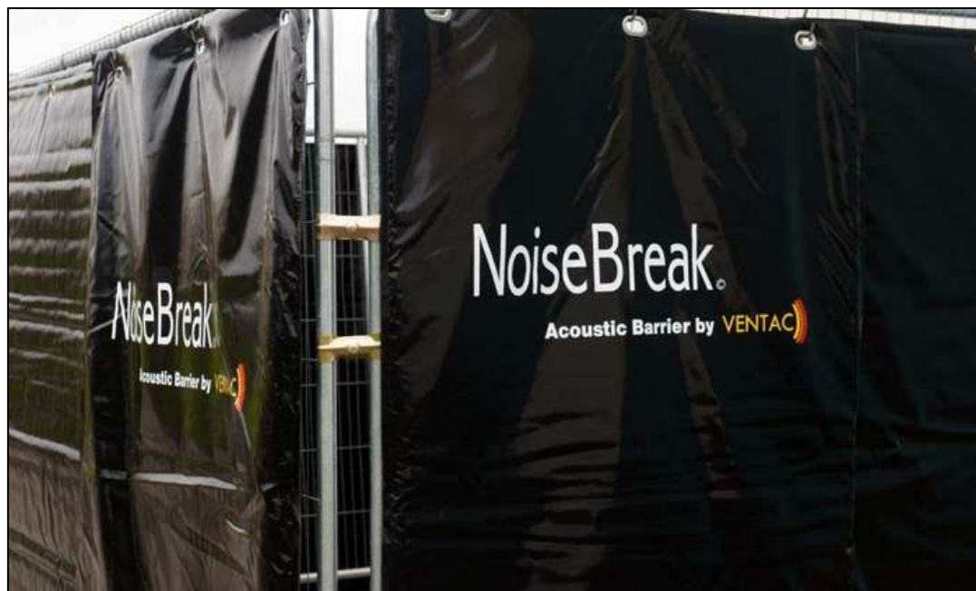
Figure 10-18: Temporary Construction Noise Barrier © Ventac
