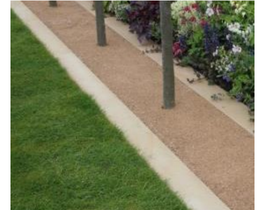
Self binding gravel edged with poured concrete strips – 120mm wide and polished
